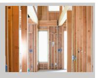
We highly recommend installing a conduit in the wall during rough in so that the electrical cable and floor sensor can be easily and quickly be drawn up during the laying of the electric heat mat.
